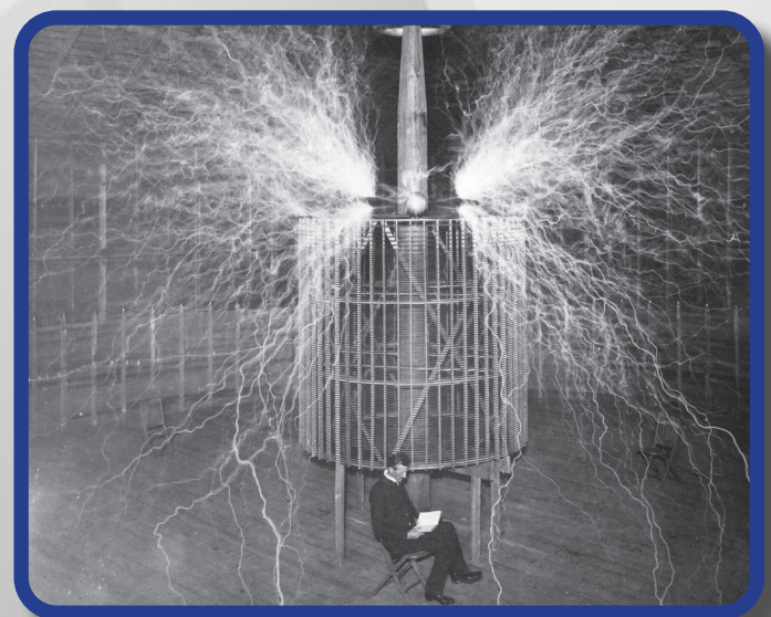
Magnifying transmitter which can generate millions of volts of electricity
