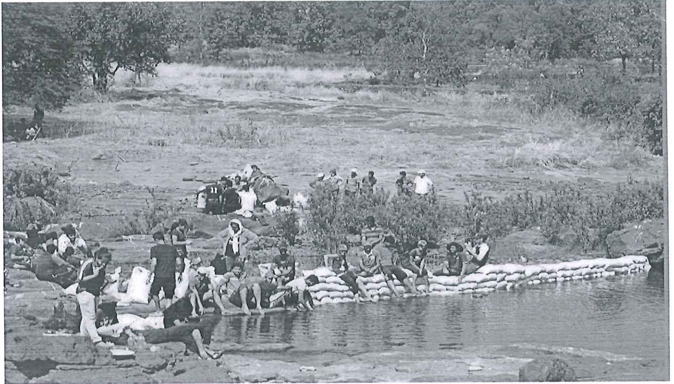
WORKING ON DAM 1
